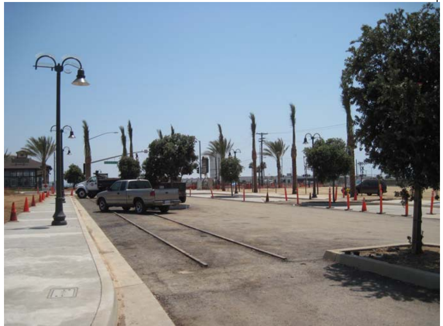
The remains of Harrison Ave. and the track that was connected to the BNSF main line look quite different than a year ago. Landscaping and new light fixtures match the look of those at the Railcar Plaza across Bay Marina Dr. Photos by Ron Sucht
