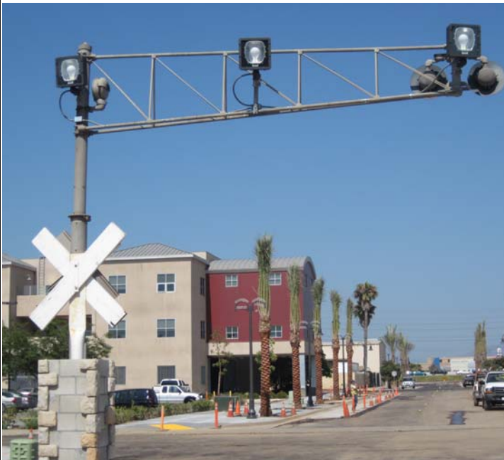
The old Cleveland Ave. crossing signal now holds spotlights on the upper arm that will illuminate the Depot at night. The concrete posts (above and right) will support the new motorized gate.
