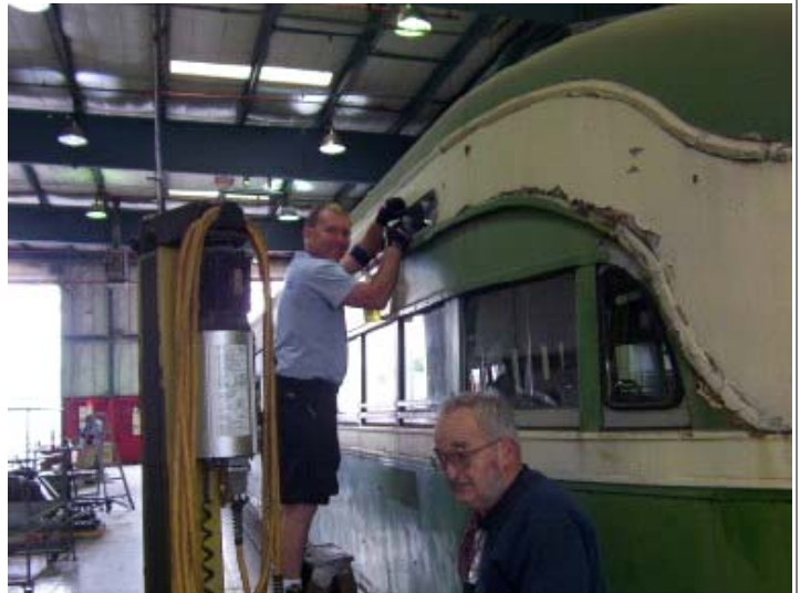
The guy on the ladder near Chuck Bencik, is Mark Delia, owner and donor of ALL of our new glass. He is installing green glasses in #529, and later #530. #531 will be glazed with #2 gray salvaged and donated by San Diego Trolley. Photo—Dave Slater
