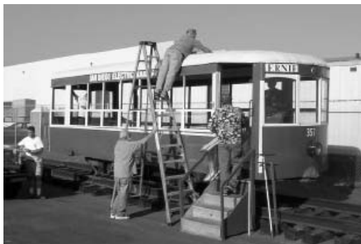
“Ernie” gets his roof patched by handy SDERA members - Photo by Dave Slater
