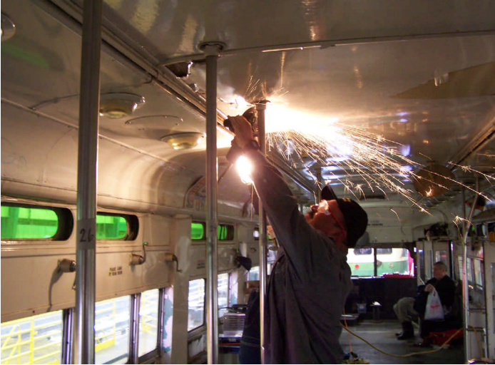
MTS Employee John Tarantino grinds away rusted in screws from the seats during the April 8th work party. - Photo by Chris Higgins
