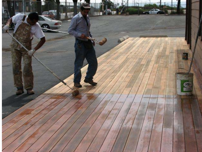
Deck stain is applied on the east side of the Depot.
